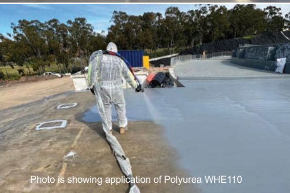
Photo is showing Polyurea WHE110 + Nitoflor PA top coat (curtain call)
