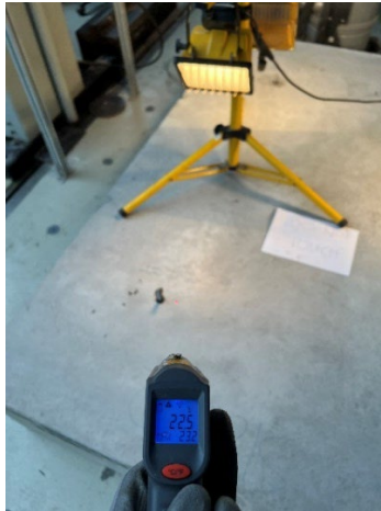
g) Heat lamps to maintain curing temperature Figure 2 Installation of anchor in concrete
