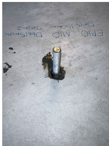
b) Anchor installed with ConbextraEP10 epoxy
