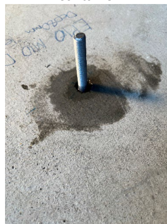
f) Anchor installed in concrete
